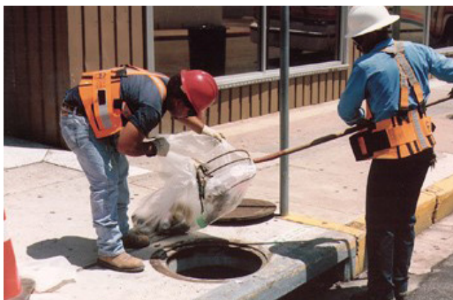
Stormwater Department crew cleaning a storm drain
